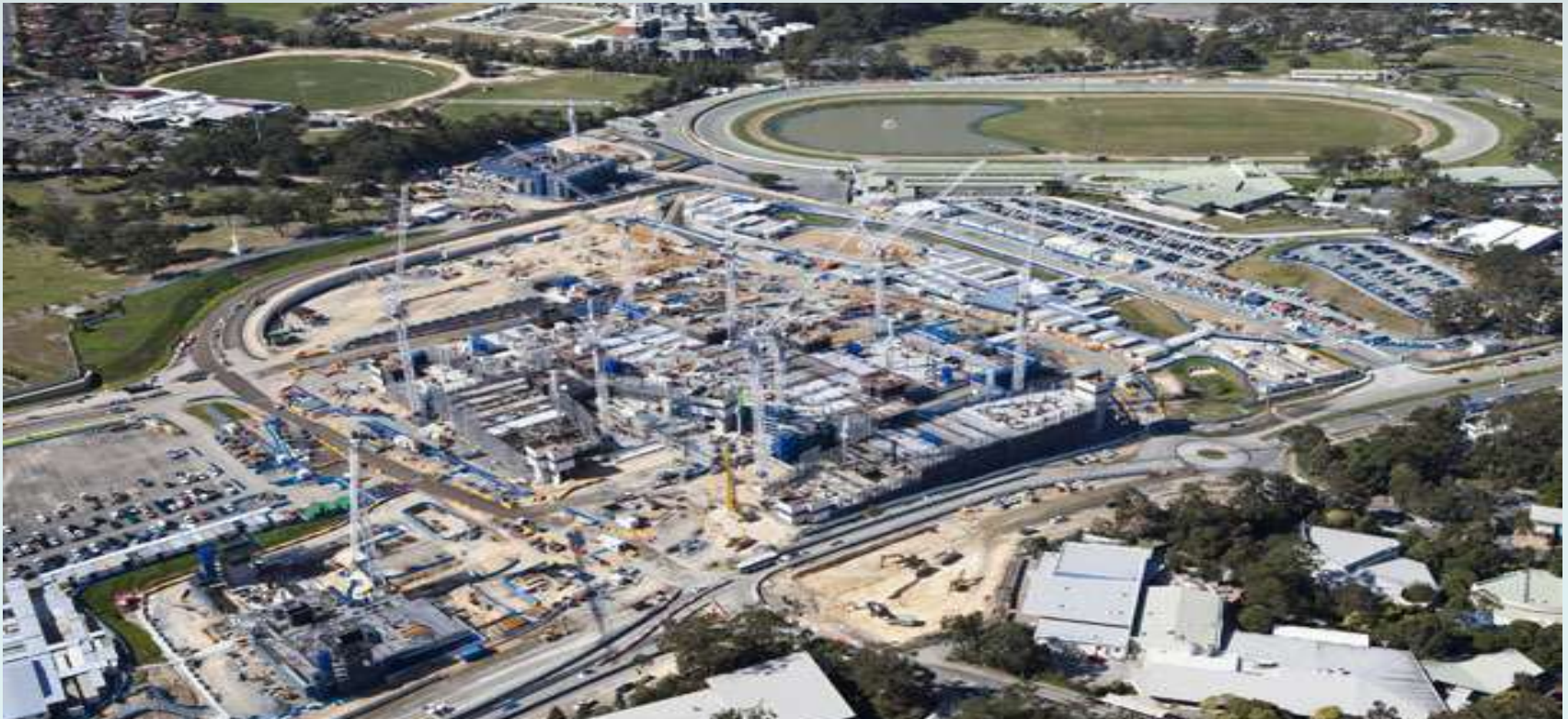
Gold Coast University Hospital Station shell construction progress (August 2010)
